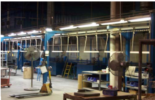
Photo of powder coating line with T8 fluorescent task lighting
