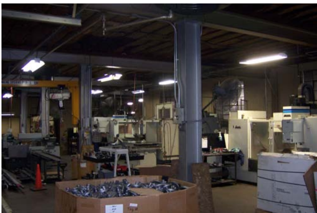
Photo of machine shop with T8 fluorescent fixtures
