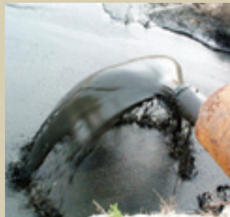
FROM LEFT TO RIGHT: DREDGING TECHNIQUES MIX PROGRESSIVELY LESS WATER WITH THE SEDIMENT. SHOWN ARE THE DISCHARGES FROM A HYDRAULIC DREDGE, A SLURRY PUMP, A CONCRETE PUMP, AND A CLAMSHELL BUCKET.
