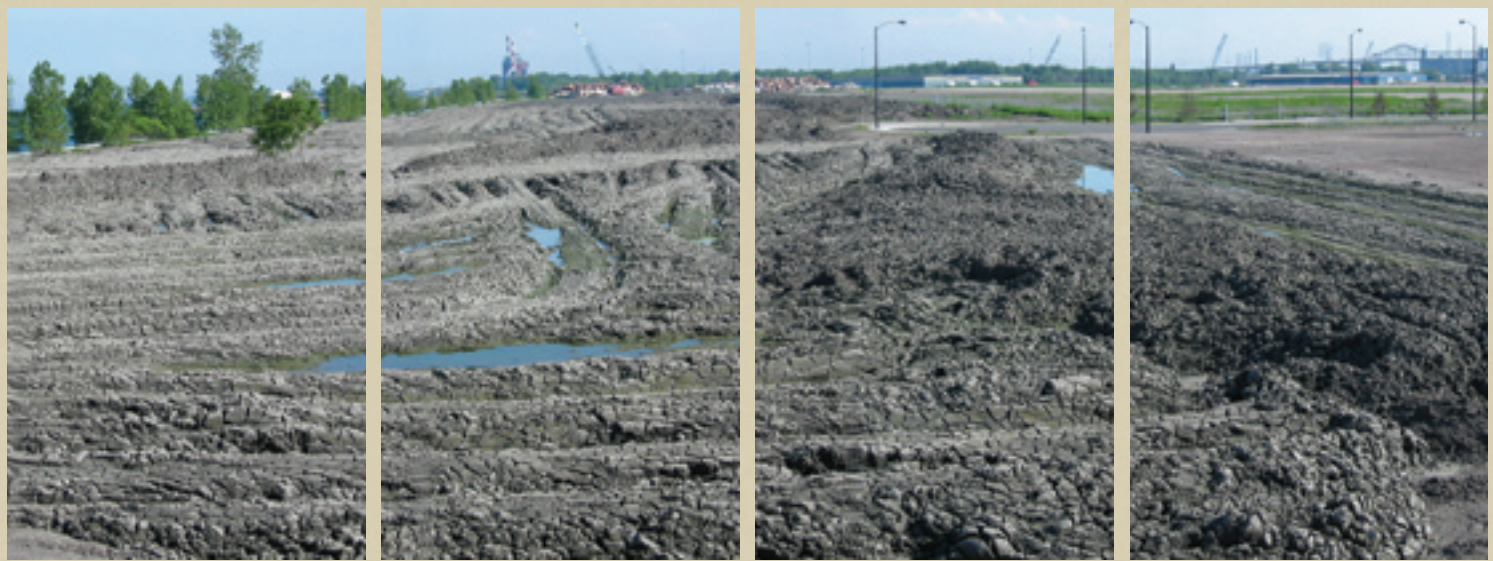
ROUGH, GRADED SEDIMENT DRIES AT THE U.S. STEEL SOUTH WORKS SITE ALONG LAKE MICHIGAN.
