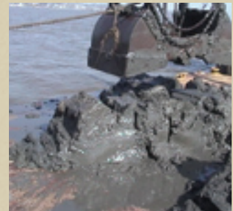
FROM LEFT TO RIGHT: DREDGING TECHNIQUES MIX PROGRESSIVELY LESS WATER WITH THE SEDIMENT. SHOWN ARE THE DISCHARGES FROM A HYDRAULIC DREDGE, A SLURRY PUMP, A CONCRETE PUMP, AND A CLAMSHELL BUCKET.
