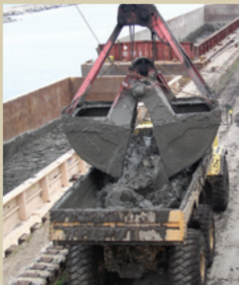
OFFLOADING BARGE ONTO TRUCK IN CHICAGO
