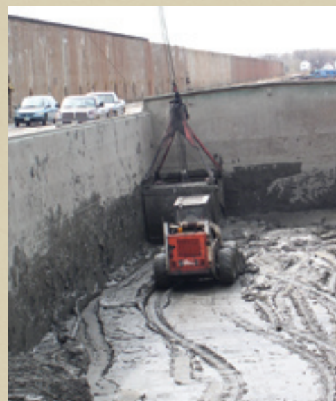
REMOVING THE LAST OF THE SEDIMENT FROM BARGE
