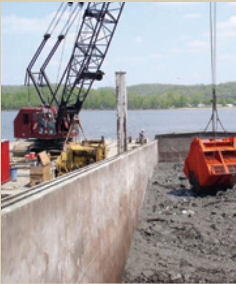
LOADING BARGE ON LOWER PEORIA LAKE IN APRIL
