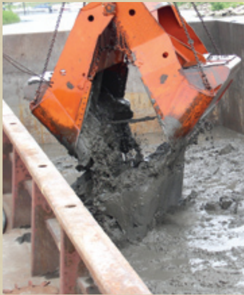
DISCHARGING FROM CLAMSHELL BUCKET
