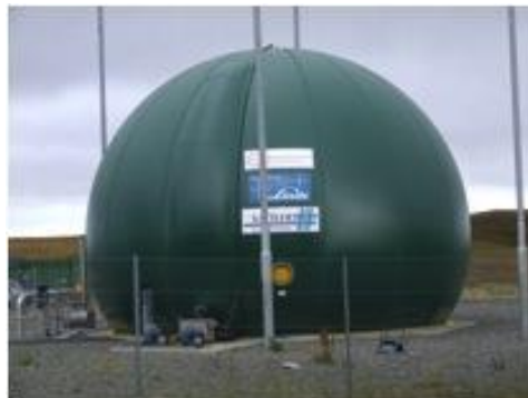
Anaerobic Digestion Methane
