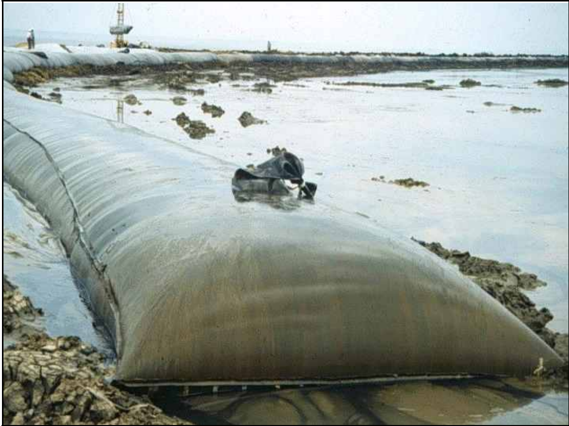
Figure 10. Geotextile tubes filled with sand and sediment are becoming increasingly popular in water resource applications. They can be used in place of riprap to protect shorelines and are capable of supporting vegetation. Tubes could be used in shallow water to break up waves. They could serve numerous functions in an Illinois River Restoration Project including protecting islands from the erosive force of waves generated by wind and vessels.
