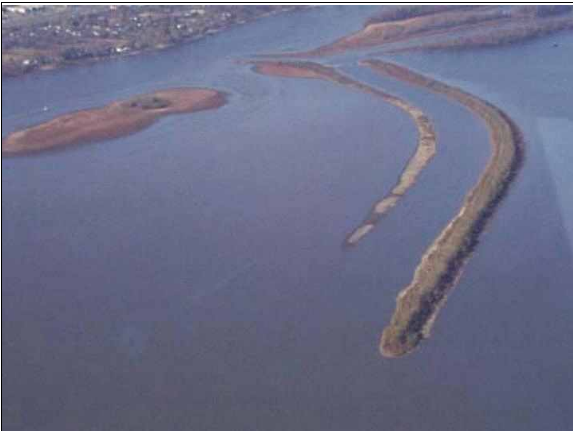
Figure 8. The two long, narrow islands in the foreground were constructed by the Corps of Engineers in 1994 as part of the Environmental Management Program. They are still in good shape after withstanding five years of waves and weathering without riprap or other protection. The islands are used extensively by numerous species, especially birds. They also break up wind fetch and reduce the adverse effect of waves.
